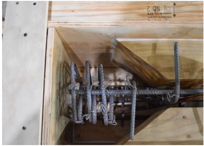
b) Stirrup arrangement at end
