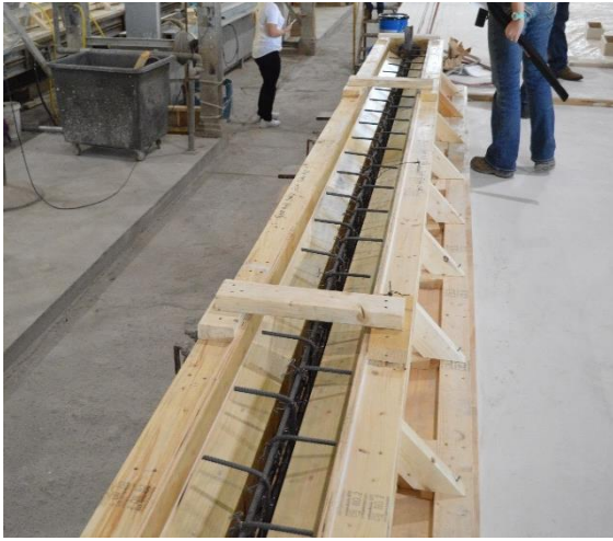
a) Formwork of the beam
