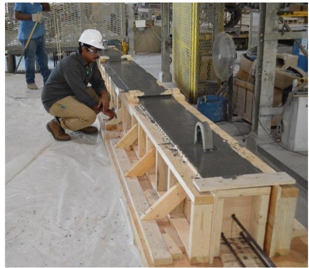
d) Beam finishing after completion of casting
